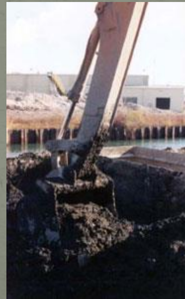
Dredging the bottom to remove accumulated pollution.
